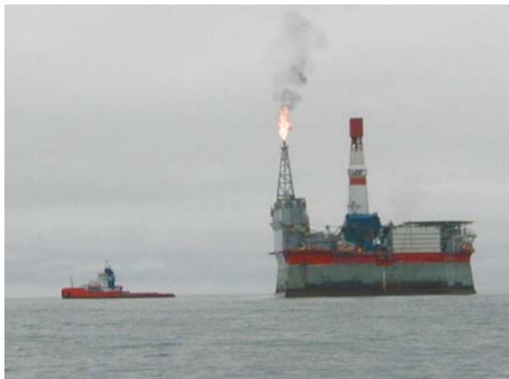
Fig. 5 Installation of the "Moliqpak" oil production platform.
